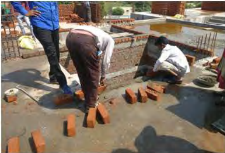
Making of the Brick Wall for the first floor.
