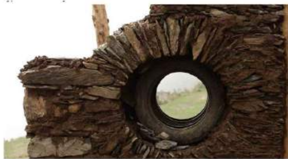
circular opening using tyre as formwork
