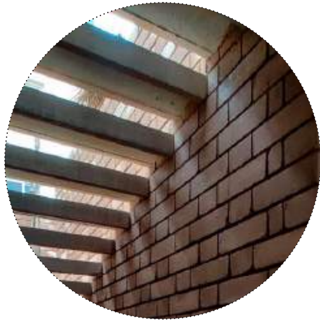
PRE CAST STAIRCASE (UNDER)
