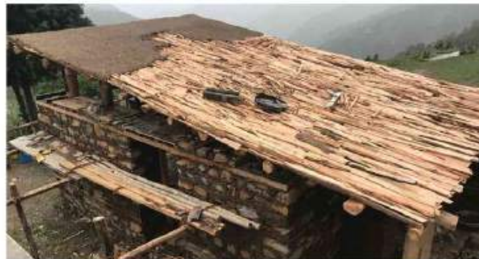
layering of roof (wooden pieces and mud)
