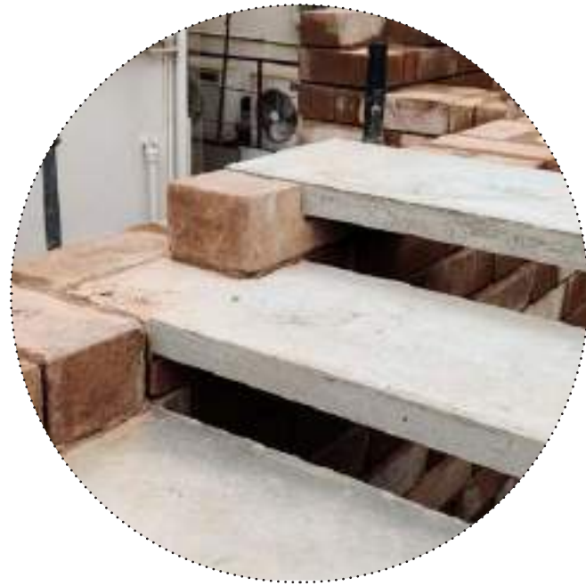
PRE CAST STAIRCASE LAYING
