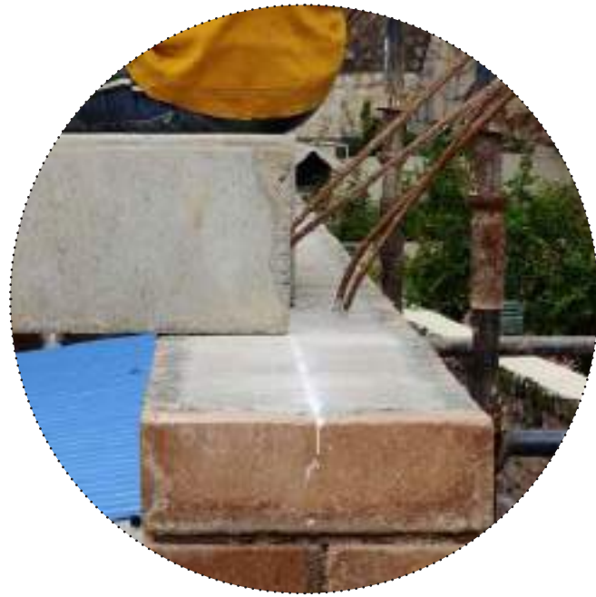
PLACEMENT TO PANEL TO MAKE ROOF
