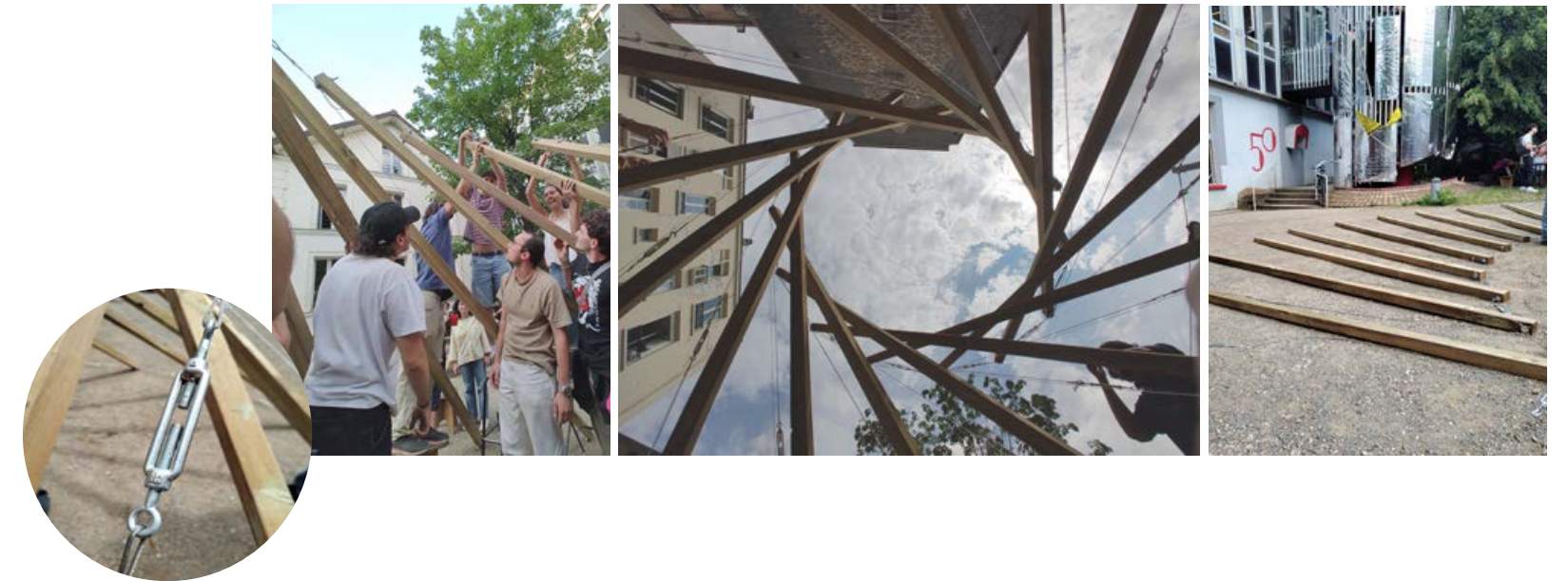
DETAIL OF TENSION CABLES
